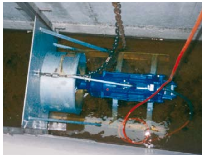
Submersible mixer in a ring channel
